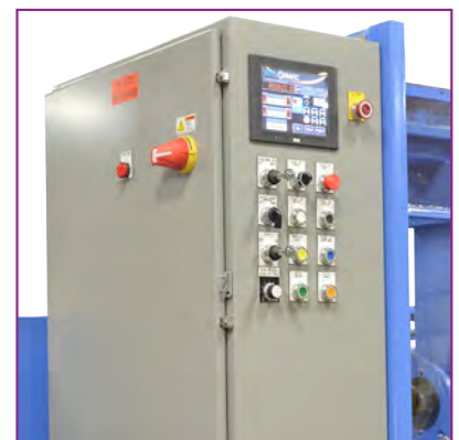
PLC with HMI and Analog Controls
