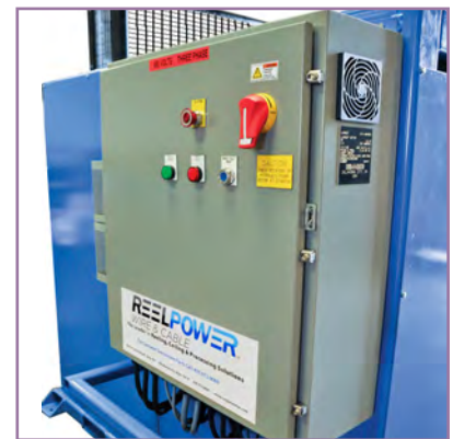
UL-508 Panel Box
