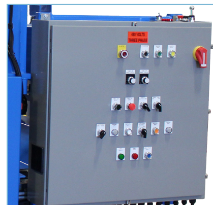
Main Control Enclosure
